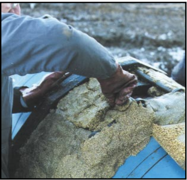
P1* application: Profiling Mastic on Tybar...
