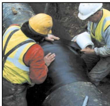
being overwrapped with Densoclad Tape...
