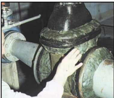
Profiling with Densyl Mastic.
