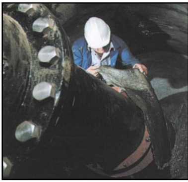
P1* application: Mastic Blanket on flange...
