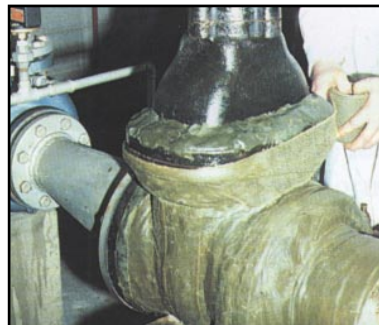
Overwrapping with Denso Tape
