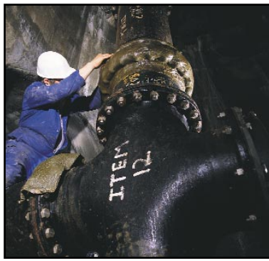
being overwrapped with Denso Tape...
