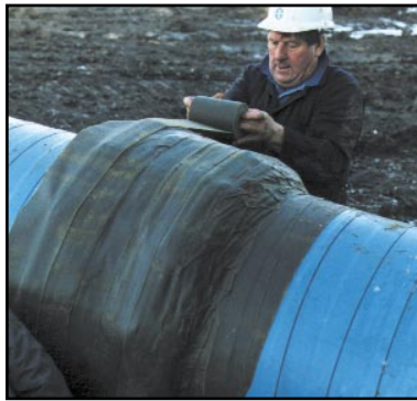
being overwrapped with Denso Tape...
