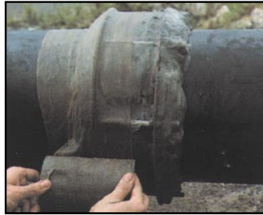
Overwrapping with Denso Tape
