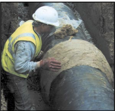
P2* application: Profiling Mastic on flange...
