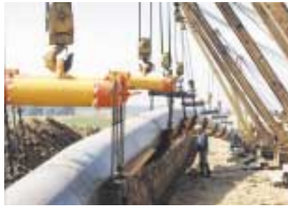
asymmetrical three-ply tapes, which are preferably used today.
