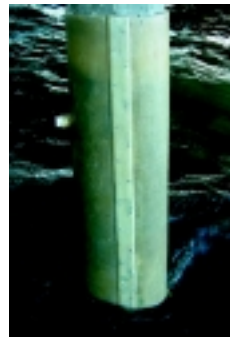
SeaShield 550 Epoxy Grout being pumped into the SeaShield Series 500 Fiber-Form Jacket.
