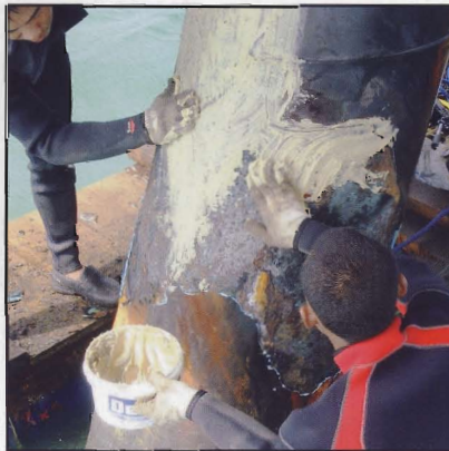
2. Denso S105 paste is then applied to the cleaned area only.
