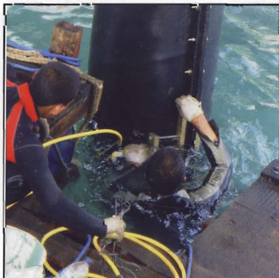
5. Finally SeaShield 2000 FD Jackets are attached using a hydraulic pump to compress the joint to enable easy bolting.
